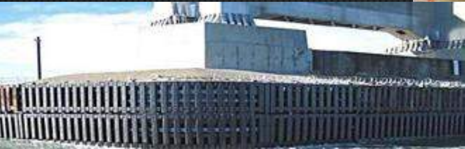
LDPE Hybrid Beams for Collision Protection of Bridge Piers & Columns (Oakland Bridge, San Diego Bridge, ..)
