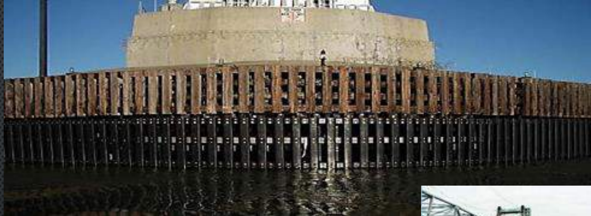
LDPE Hybrid Beams for Collision Protection of Bridge Piers & Columns (Oakland Bridge, San Diego Bridge, ..)
