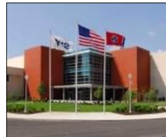
Y-12 National Security Complex
